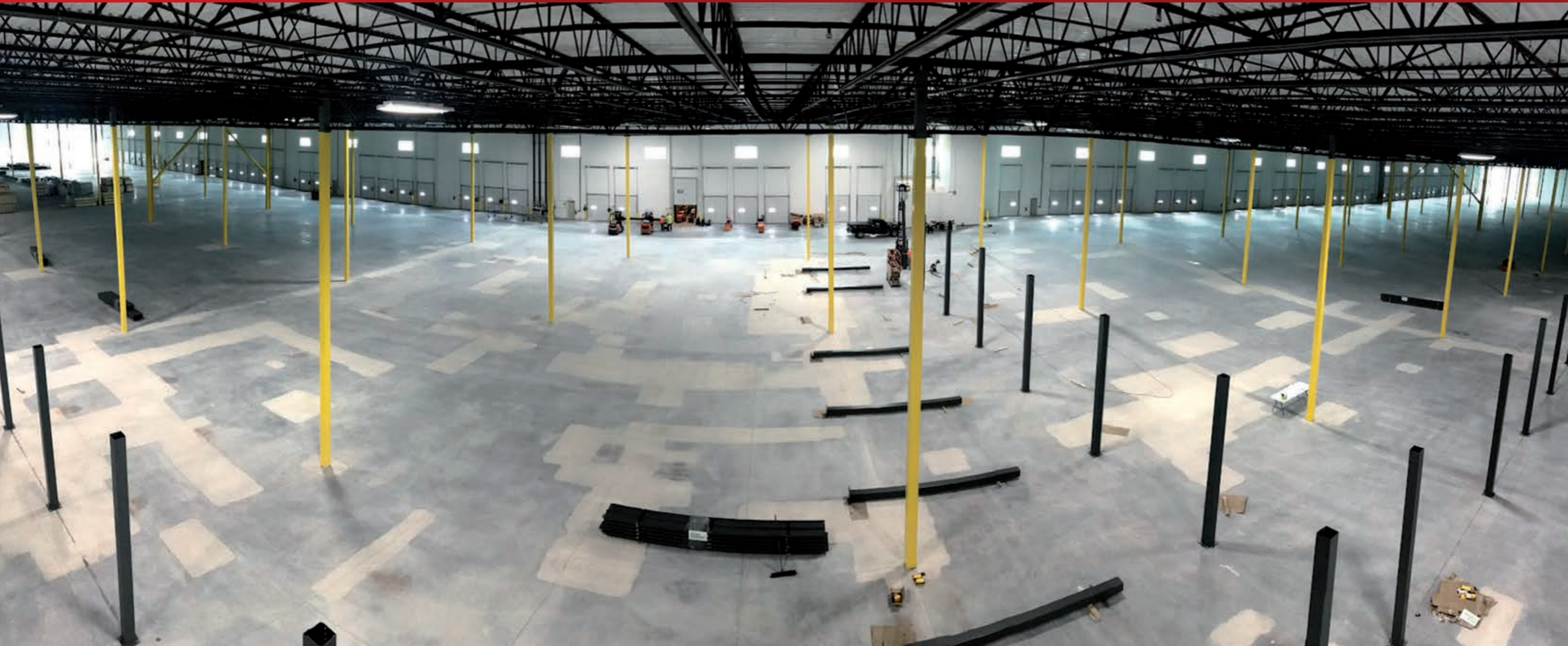
Floor ground into compliance for automated warehouse.
